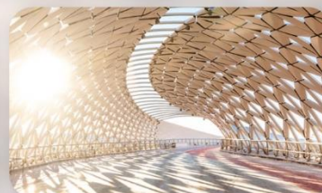
Atyrau Bridge Astana
